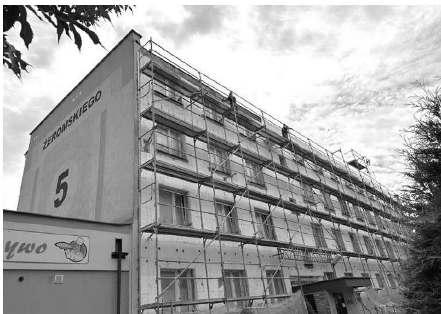
Fig. 26. Thermal modernization works on the building at 5 Zeromskiego Street in Lomza
