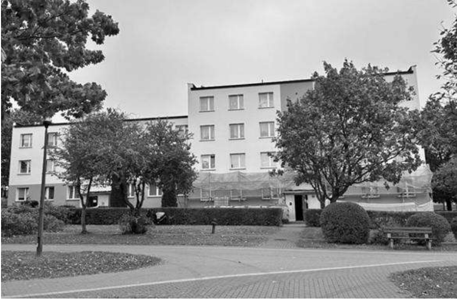
Fig. 27. Façade of the building at 5 Zeromskiego Street in Lomza
